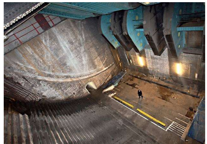
Fig 9 Bascule Chamber, Radius 15 m
