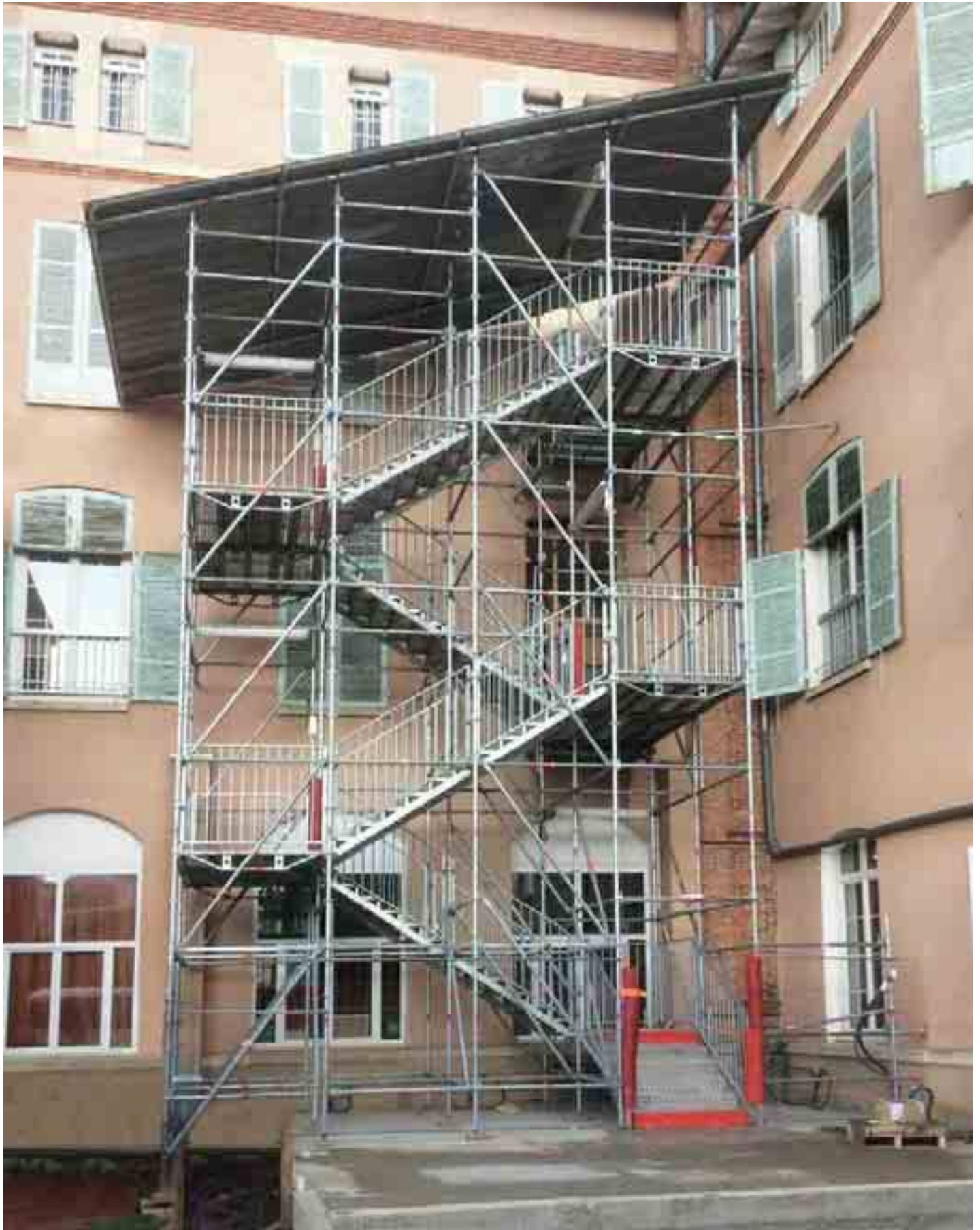
Escalier Public - Everest Echafaudages
